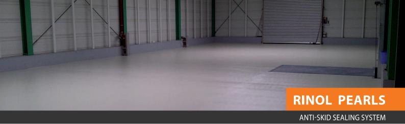
Two- layer epoxy resin sealing system for concrete and similar substrates. Slip resistance is achieved by adding RINOL Pearls. 0.5 mm to 0.8 mm layer thickness
