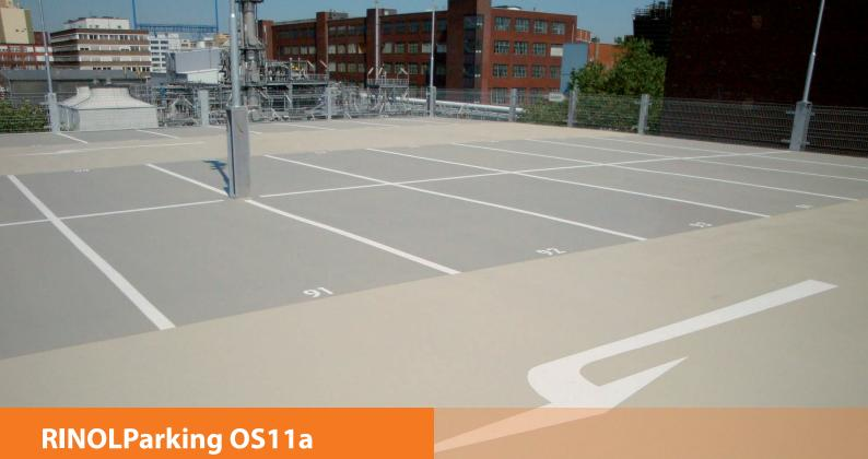
Elastic multi-storey car park coating for heavily mechanically stressed surfaces suitable for traffic according to the "Directives for the protection and repair of concrete structures of the German Reinforced Concrete Committee" DIN EN 1504:2
